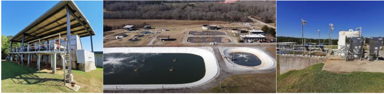
Figure 8 – Pendleton-Clemson Regional Wastewater Treatment Plant Upgrade (existing facilities)
