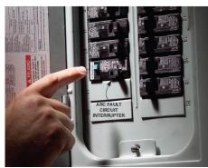
What To Look For: Outlet or wall is warm to the touch; outlet is discolored; circuit breakers frequently trip, or fuses frequently blow; a burnt smell of insulation is noticeable.
