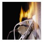
Extension cords can be used for up to 90 days but must be used properly. Surge protectors are recommended over power strips and extension cords. However, a sufficient number of well located three-wire/grounded outlets will eliminate the need for extension cords or power strips.
