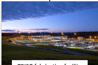
TRISO fabrication facility
