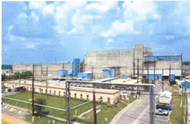
Photo: Aging H-Canyon reprocessing plant, built in the early 1950s; DOE’s last such reprocessing facility. A number of equipment and operational issues have recently plagued the facility, raising concern that it should be closed before a serious accident takes place.
