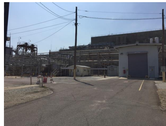
Loading Station and Blend Tanks
