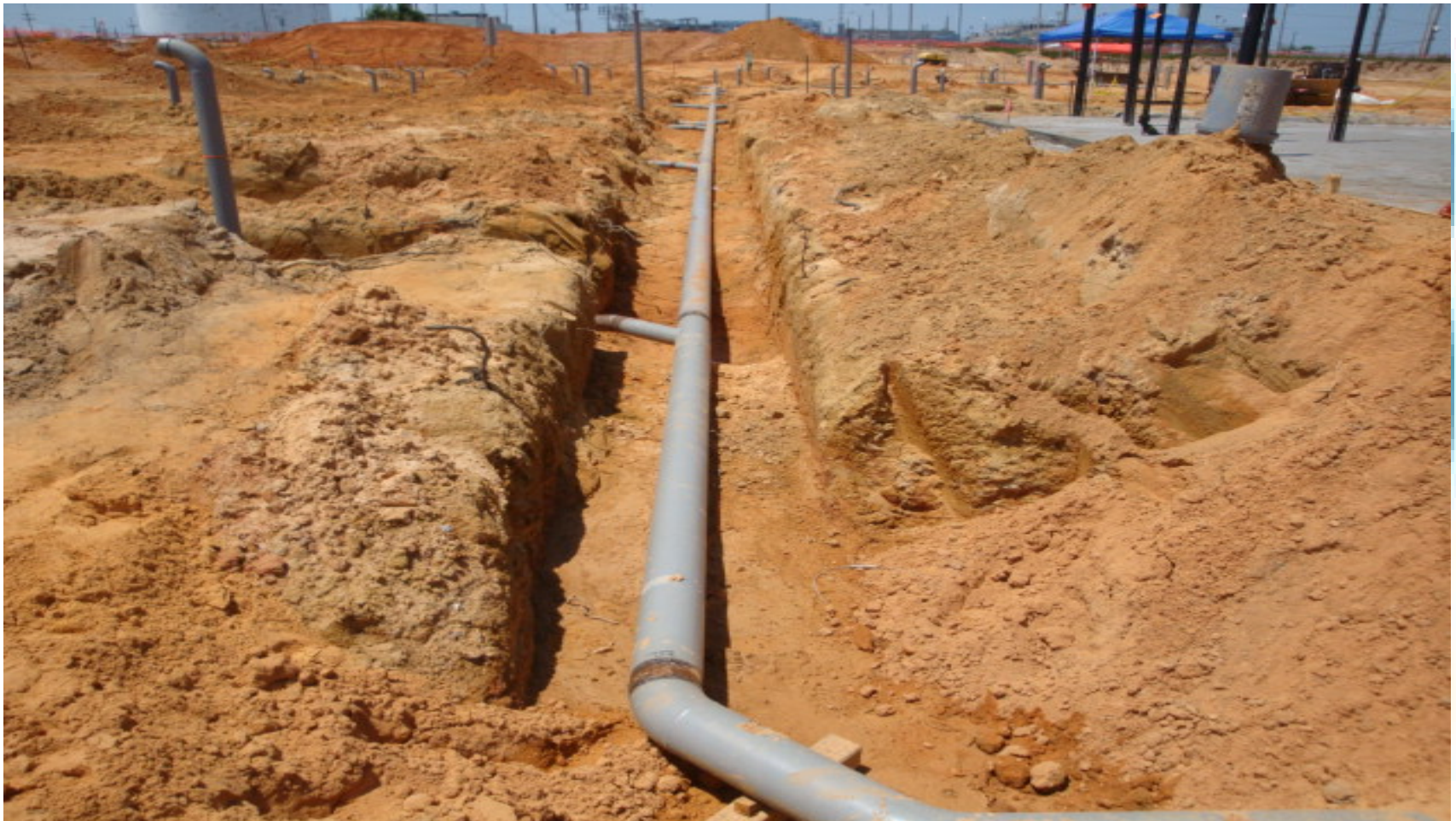
WSB Process Drain Underslab Piping
