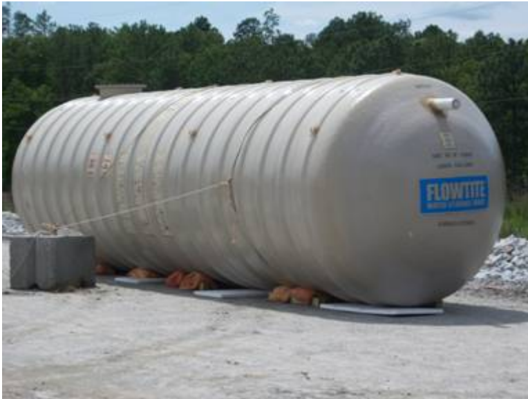
Installation of MOX Administration Building Rain Water Collection Tank
