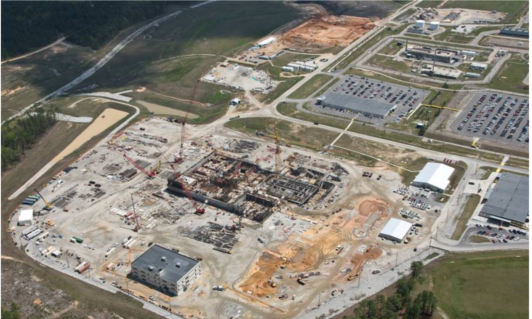
MOX Construction Site April 2009
