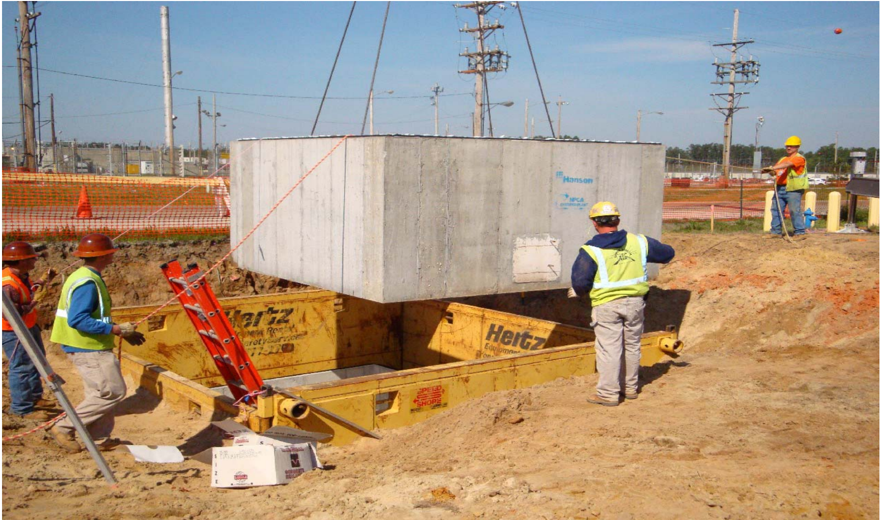
WSB Electrical Manhole Installation
