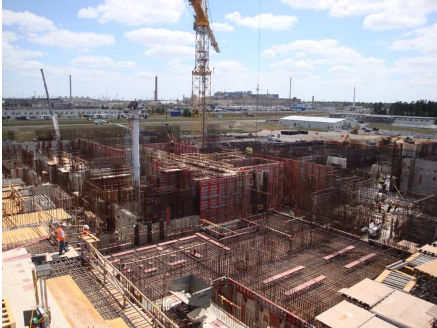
MFFF Looking South West - May 2009
