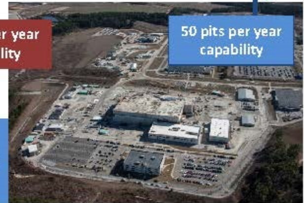
Savannah River Site
