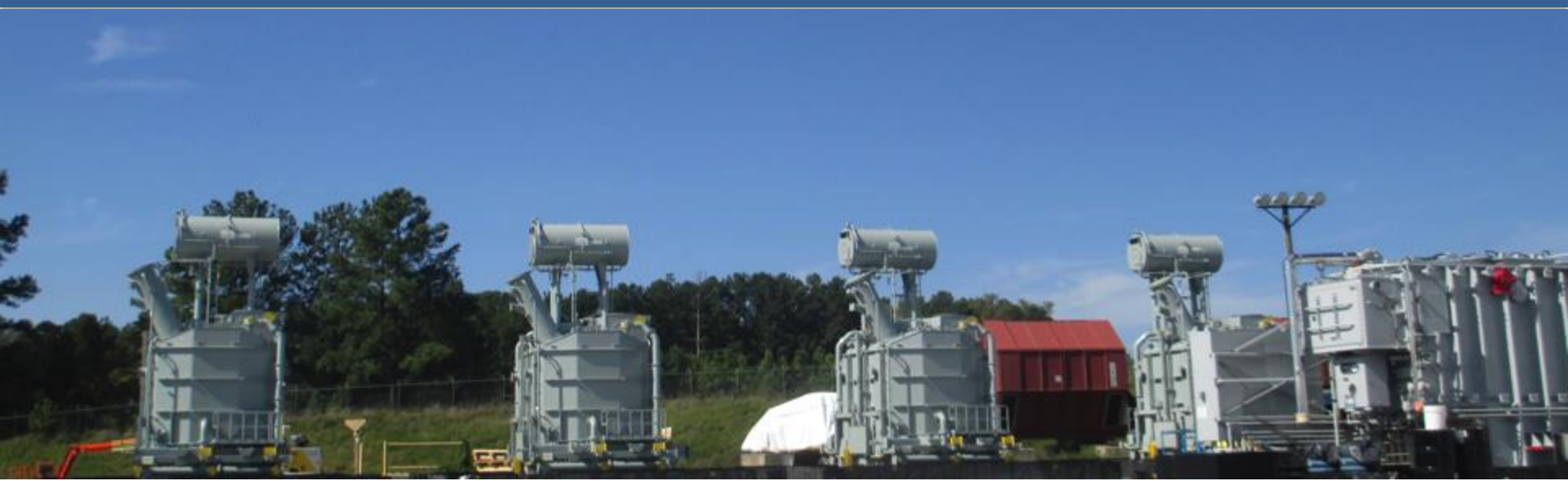
Oil Filled Transformers
