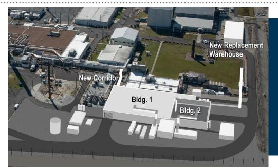
Replaces 1950s vintage H-Area Old Manufacturing (HAOM) facility - oldest and largest Tritium process facility – Assembly, final inspection, and packaging processes
