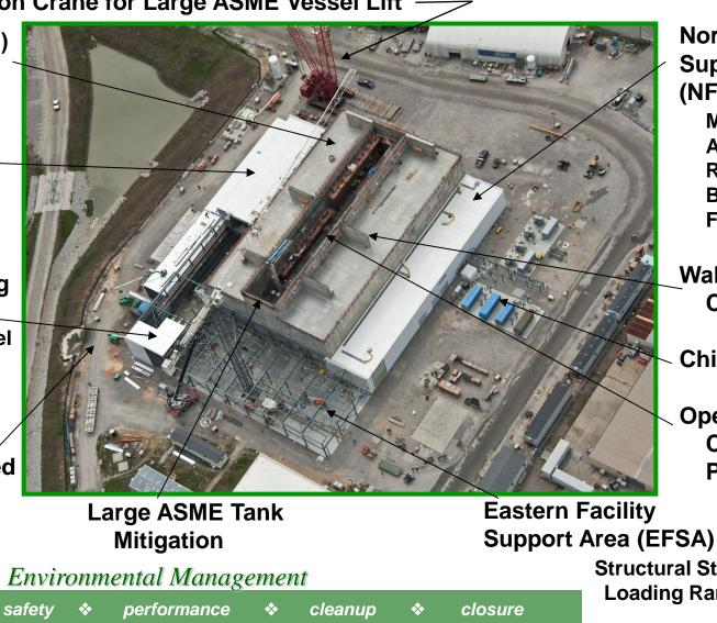
**North Facility** Support Area (NFSA) MCCs Set **Air Handlers Set Roof / Siding Bus Supports Fire Proofing**
