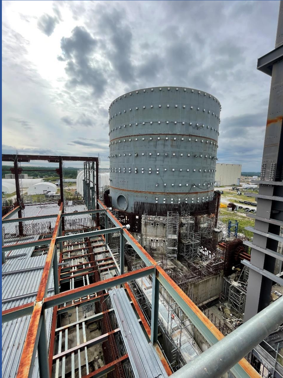
Additional view of Reactor 2 Containment Structure
