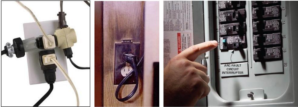
What To Look For: Outlet or wall is warm to the touch; outlet is discolored; circuit breakers frequently trip, or fuses frequently blow; a burnt smell of insulation is noticeable.
