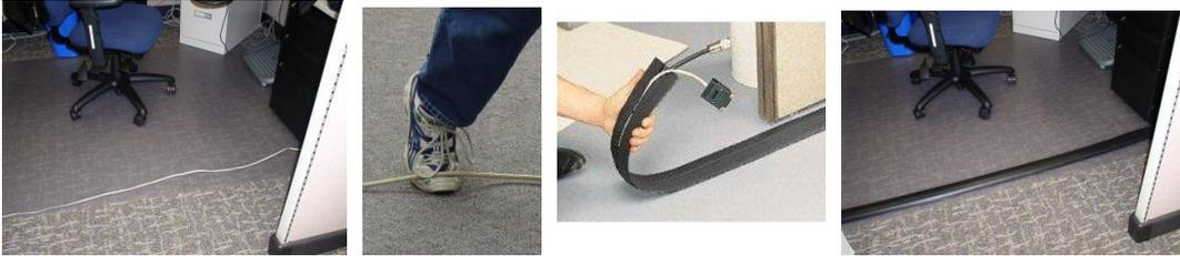
Remedy: Keep extension cords away from foot traffic and doorways to prevent damage to the cords as well as a tripping hazard. To help prevent tripping, tape down or cover the extension cord with a cable cover, or rearrange office furniture. Better yet, add more outlets to eliminate the need for an extension cord.
