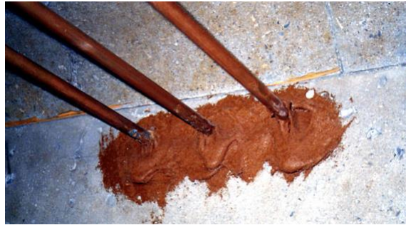
Intumescent caulk around copper pipe penetration
