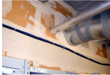
Sheetrock and joint compound
