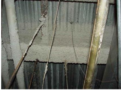
Sprayed on fireproofing
