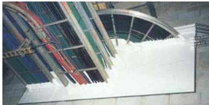
Penetration Fire Seal membrane - http://www.fire-stopsystems.com/elastaseal.html
